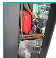
Expansion vessel, flue gas exhaust fan
