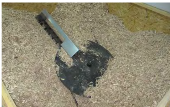
Wood chips storage with the mixer connected to the transporter
