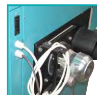
Flue gases exhaust fan, connector for the pump and sensor
