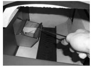
Cleaning of combustion chamber with fire hook
